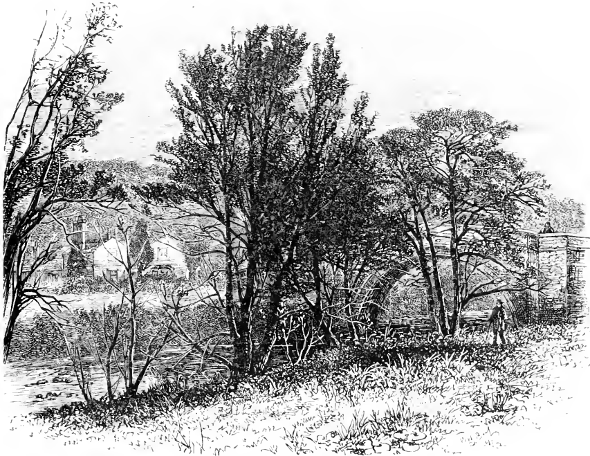
Edensor Mill Lodge and Beoley Bridge.
